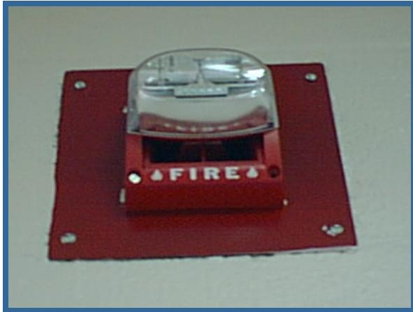
Fire horns and strobe lights are activated when the fire alarm panel is activated.
